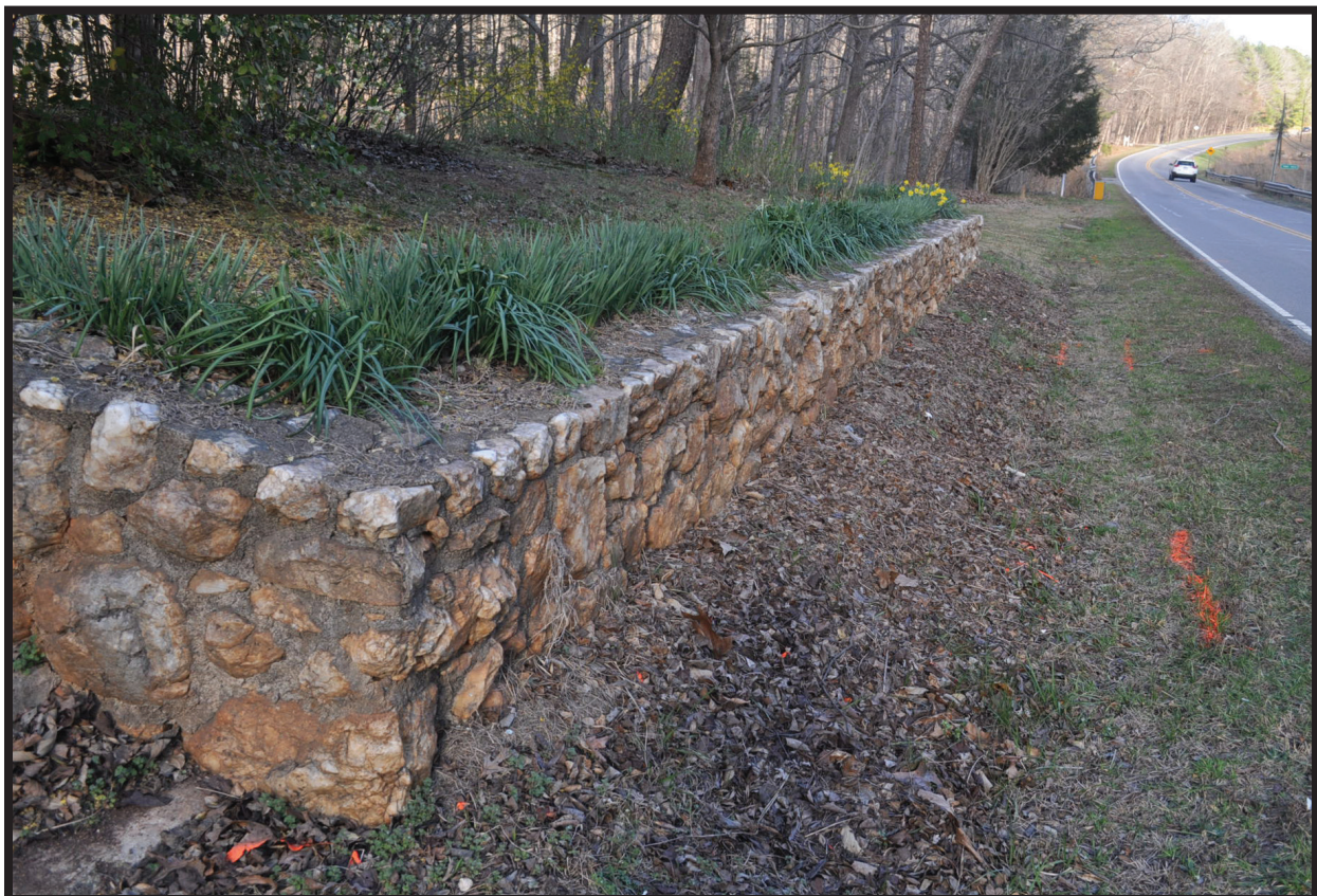
Figure 4. Quartz Retaining Wall
