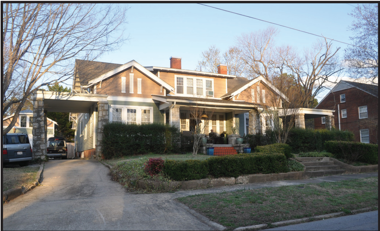
Figure 24. Hancock-Easton House, Oxford
