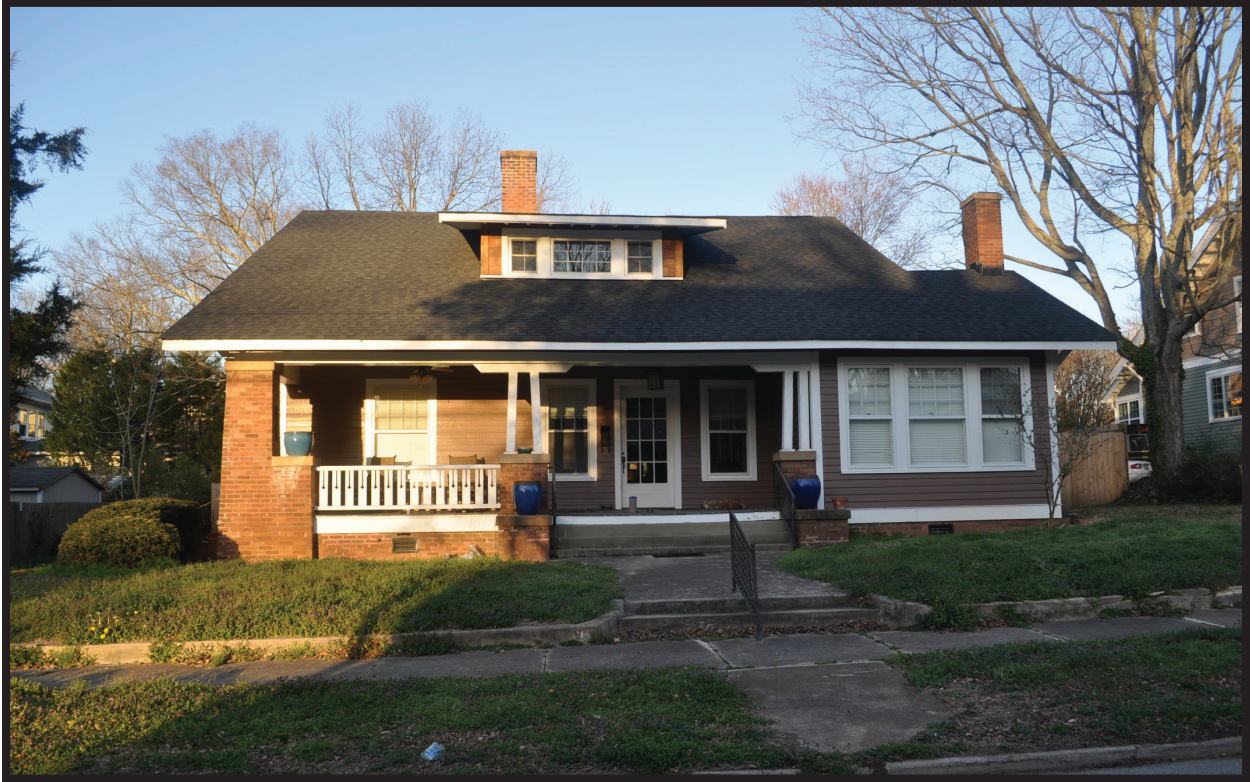
Figure 23. 407 Hancock Street, Oxford
