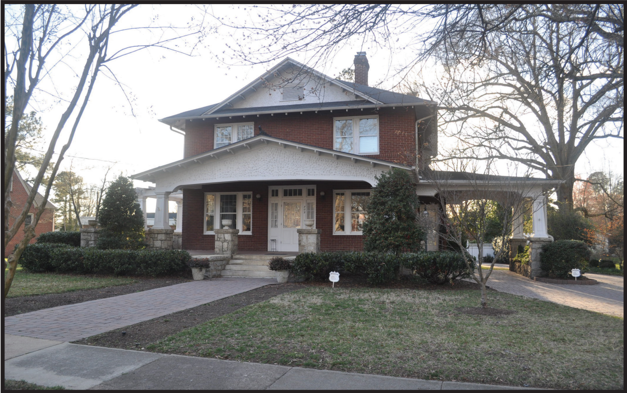
Figure 21. Crews-Turner House, Oxford
